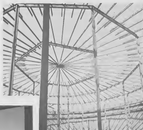
SUPPORT IN the form of I beams, common in the building trade, is needed to bear the weight of heavy steel plates for a round storage tank roof. AGUANTE DEN forma di balkinan den forma di I, común den construcion, ta necesario pa carga e peso di plachi di ataal piñá pa dak di un tanki rondó.
